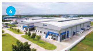
SAM Precision (Thailand) Limited (Chonburi Province) - Buildings 1 & 2
