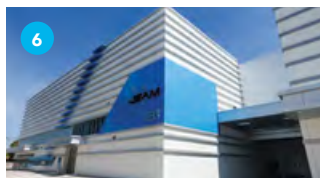
SAM Precision (Thailand) Limited (Chonburi Province) - Building 3
